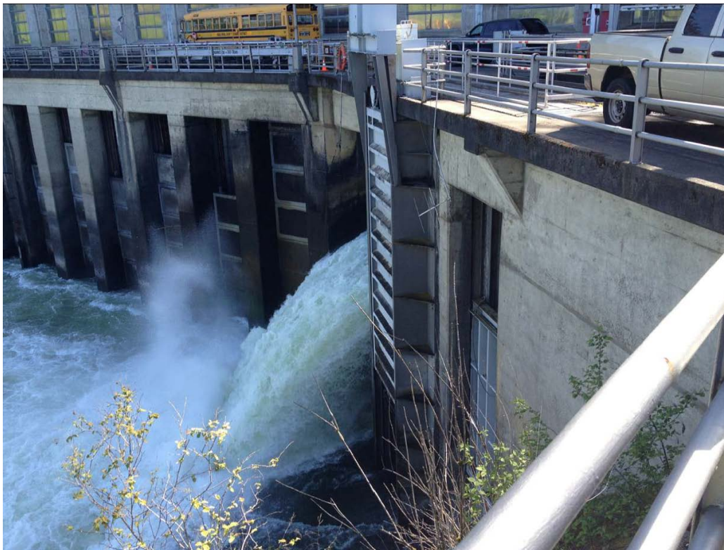
Figure 6-4. B1 ITS Outfall Pass-Thru Antenna
