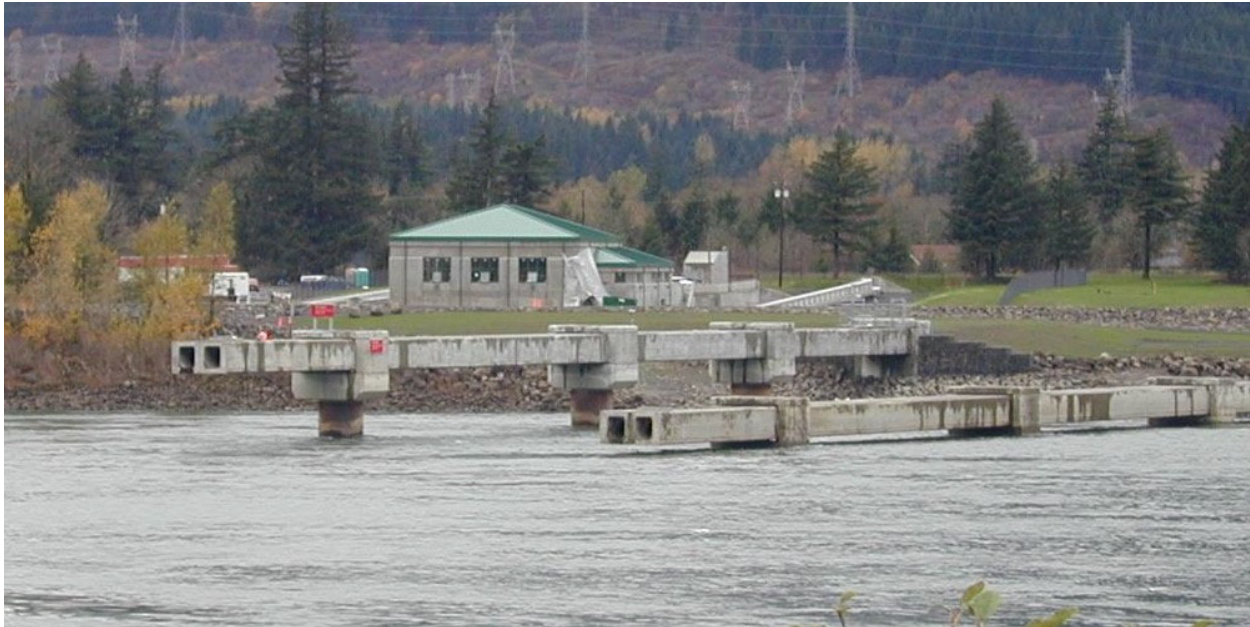
Figure 6-10. JBS Outfall Piers
